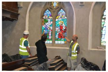
The work involved removal of the modern plaster on both side walls and its replacement with a Victorian style plaster thereby restoring the original appearance and texture of the 1870s. This type of plaster is far more resistant to damp than modern materials: Victorians were used to living in damper conditions than we would tolerate
