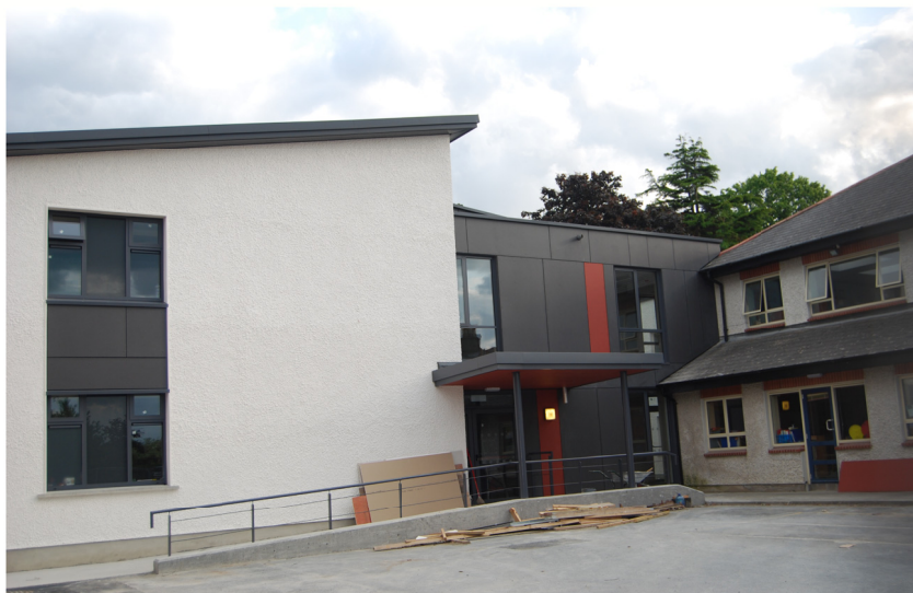
The School extension almost ready for occupation.
